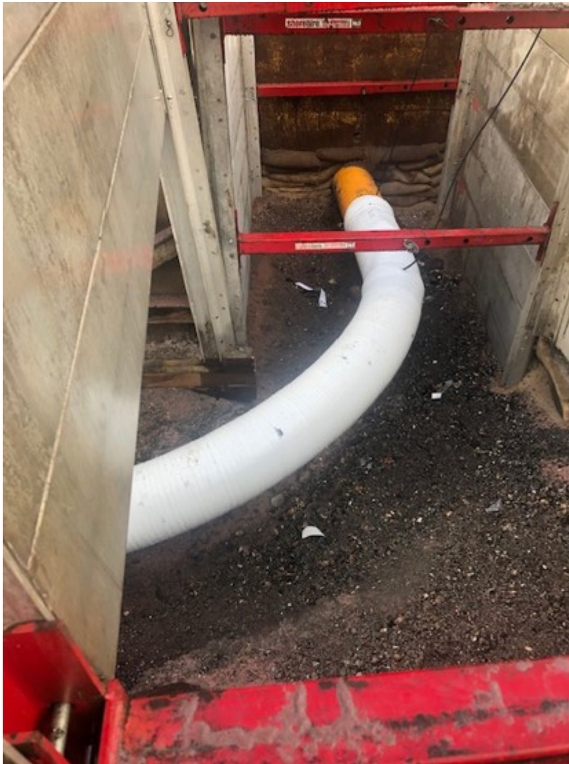
Figure 4.3 5 times diameter hot rolled induction bend installed with corrosion protection wrapping installed prior to backfill
